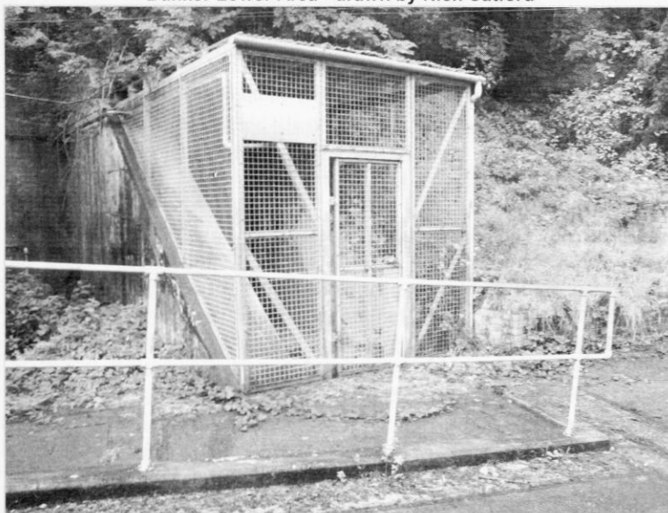
The 'dirty' entrance into the bunker - Photo by Nick Catford
